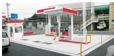
A compact self-service station, which keeps down the installation and operating costs through its compact design and limited product lineup
