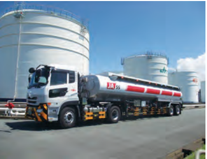
Fuel oil is distributed from seven petroleum facilities across Japan to about 2,600 JA-SS service stations.
