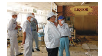
Touring a damaged JA Okayama-Nishi facility
