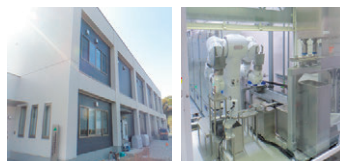
New testing building Robotic testing equipment
